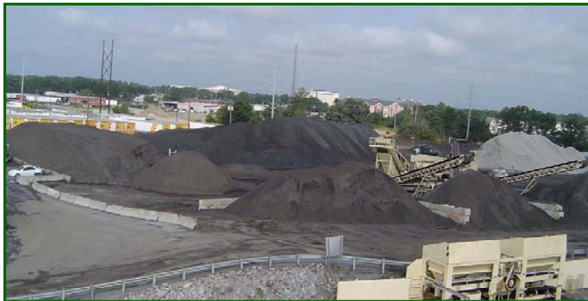
Recycled Asphalt Pavement Stockpiles (Charleston, SC)
