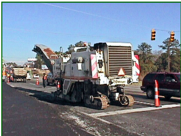
Milling Asphalt Pavement for Recycling (from SCDOT)
