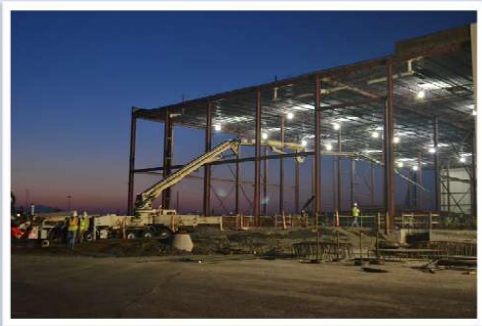
Concrete pour for the Restoration Institute Wind Turbine Test Facility being developed on the Restoration Institute campus in North Charleston. The facility will be instrumental in testing wind turbine technologies to supply alternative energy to support urban growth. This is relevant to research at the Urban Ecology & Restoration Center of Economic Excellence.
