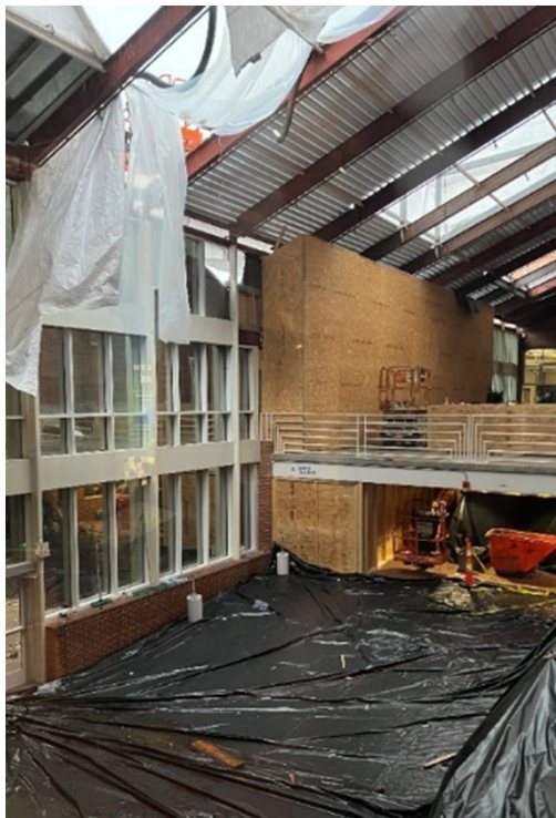
View of the Atrium roof and window replacement project
