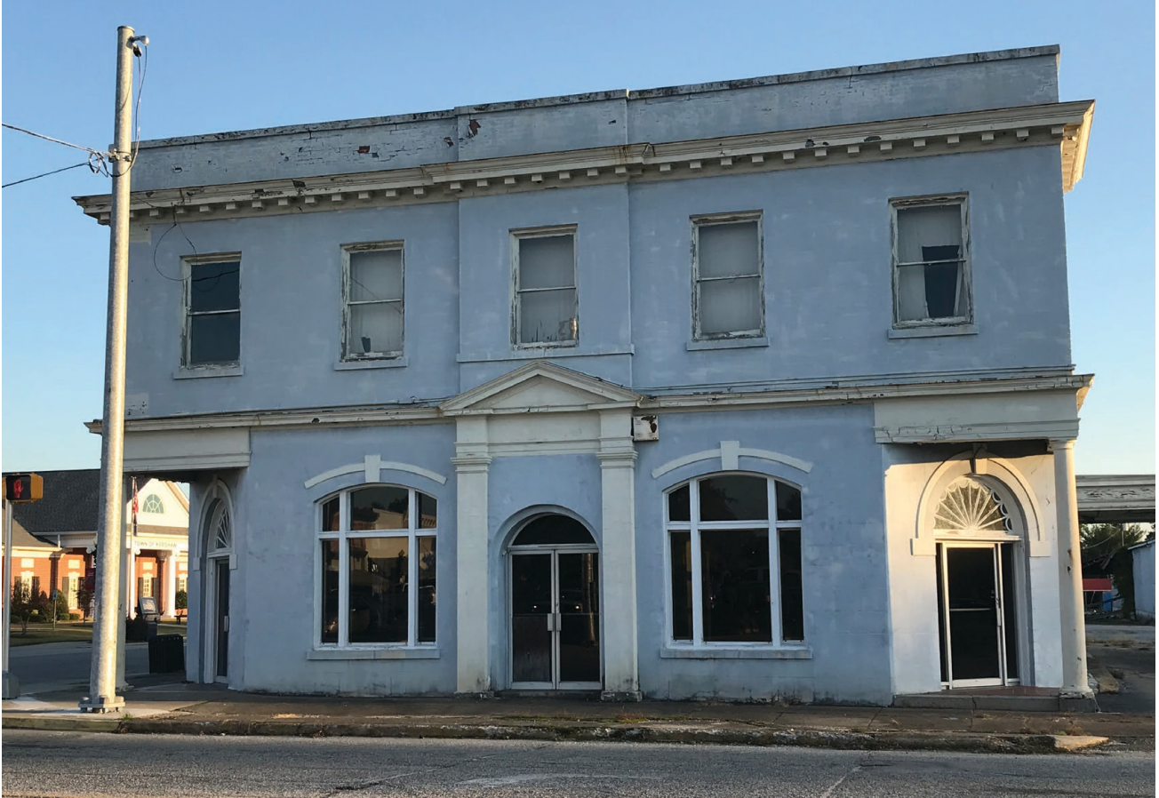
The former Bank of Kershaw building will soon house the only licensed child care center in town.
