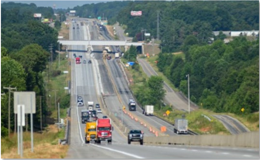
I-85 northbound lane opening
